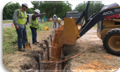
Crew completing underground rehab
