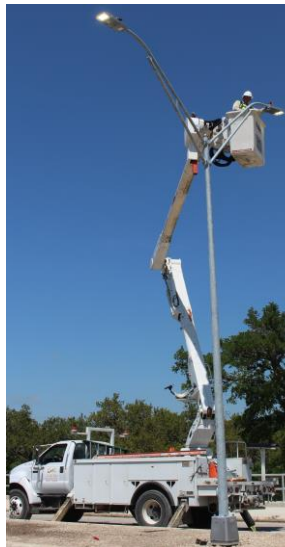
Crew working on streetlight
