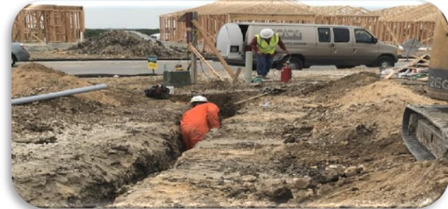
Crew completing joint trench work
