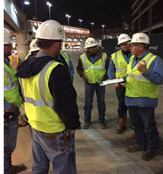
Underground Construction & Maintenance Crew
